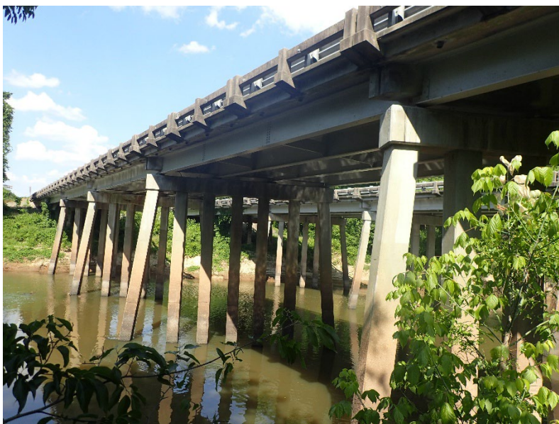
Figure 2. I-95 Bridge No. 000000001010082 on I-95 over Black Creek
