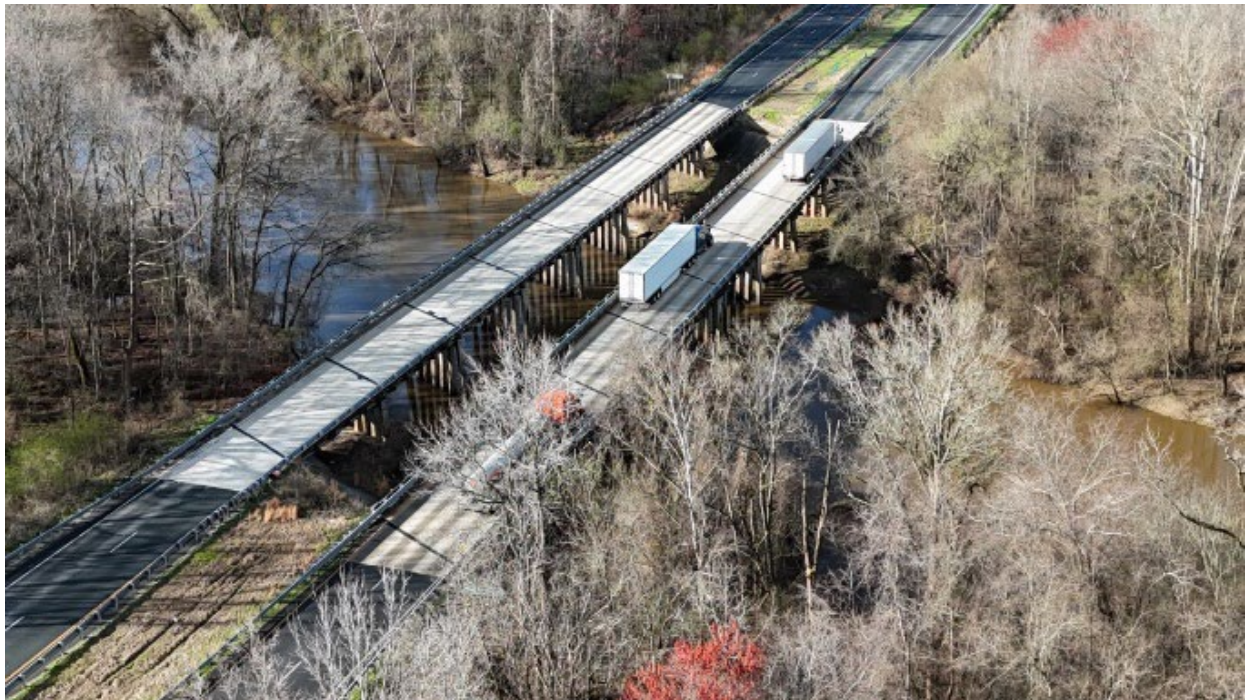
Figure 9. Neuse River Bridges
